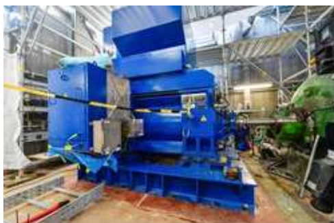
Fig. 21. Motor (L) - Compressor (R) after replacement
