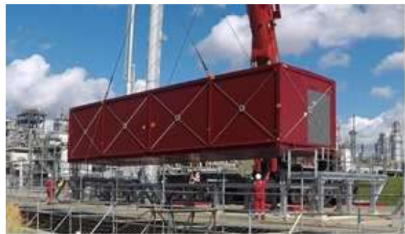
Fig. 18. Substation Module Lift
