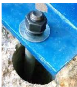
Fig. 19. Replacement of the anchoring tie-rods
