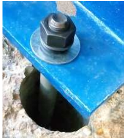
Fig. 19. Replacement of the anchoring tie-rods
