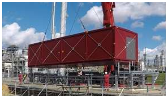
Fig. 18. Substation Module Lift
