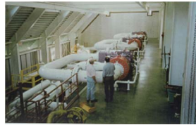
Fig. 8 Pipeline Station in US using 4 Integrated Compression Units of 3.4MW @ 10 000 rpm [5]
