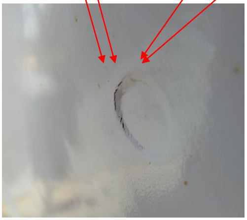
Ex"p" box lost due to bad welding
