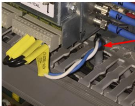
Spurious trip due to a bad cable shield assembly
