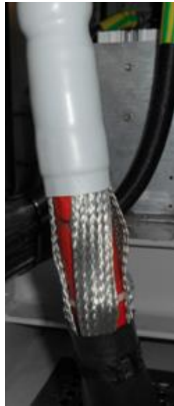
Kind of Repair
