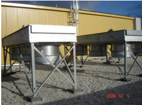
Installation of outdoor fin fan air cooler
