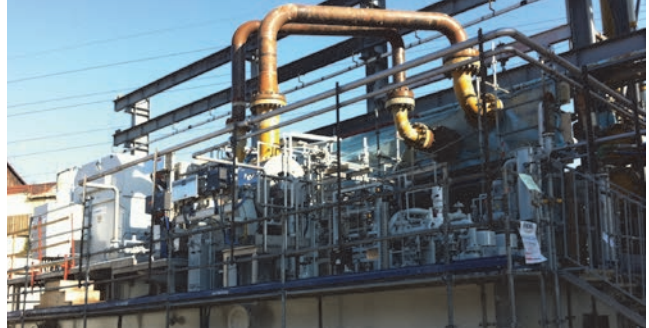
Fig.1: Moto-compressor string test arrangement
