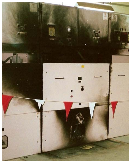
4 VCB disintegrated
