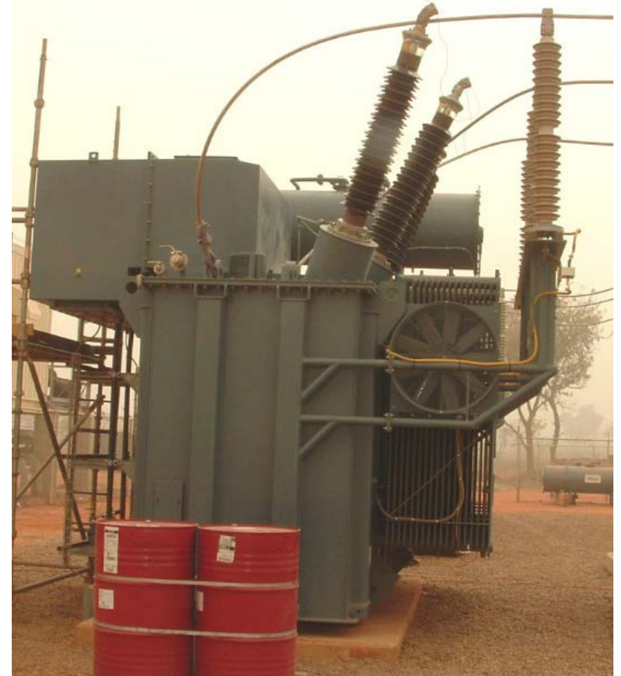
Best arrestor location – also connect arrestors before bushings
