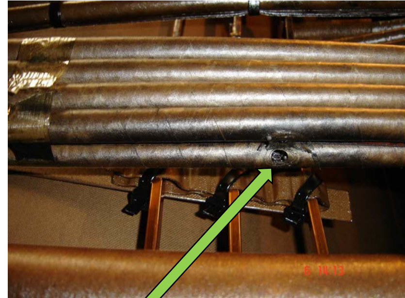
Insulation punctured
