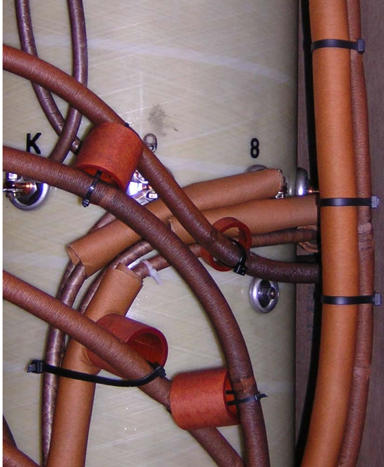
Partial discharge in regulation winding Reason for first fault
